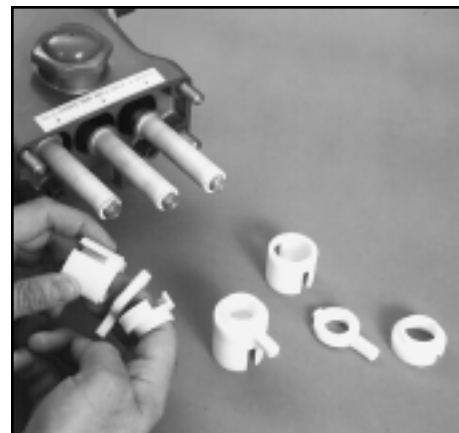
Removal of Seal Retainers and Wicks
